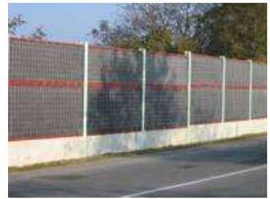
Sound protection wall • Brno
